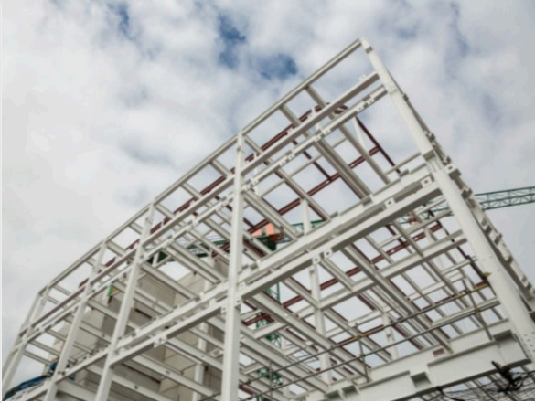
Framework of a high-rise building
